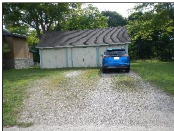
Image 6: Disturbed Gravel Driveway Area (Facing SE)
