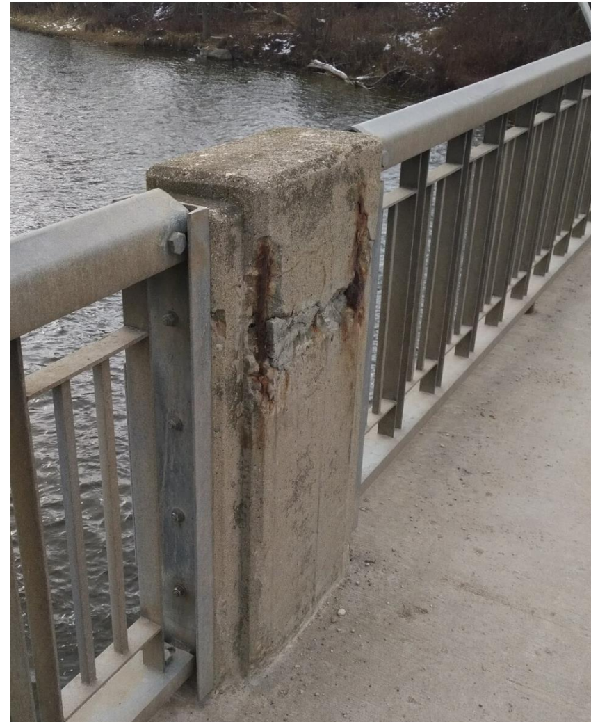
Concrete deterioration
